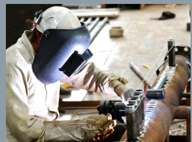
Welding of Headers
