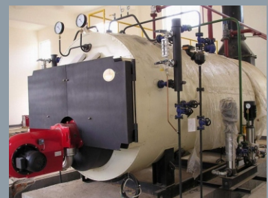
Smoke Tube Boiler
